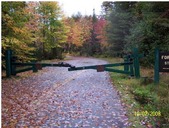
The water has undermined the gate and there is not the standard park sign on the pole out front. A new entrance needs to be designed and constructed, which might include new pavement over the existing surface treated gravel that constitutes the driveway to the parking lot. The parking lot has paved drive lanes but the parking spaces are on gravel. Some vandalism occurs, as in vehicles pushing on the gate across the service road, etc. Snowmobiles running up and down the timber
