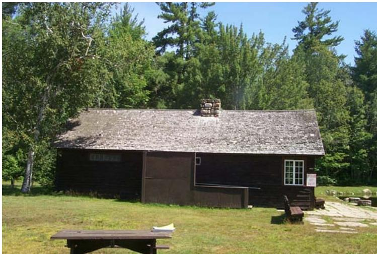
into swimming area while bypassing remainder, Bathhouse by the pool is poor and should be replaced. Observation: Recommend removing structure leaving stone fireplace, and construction new building to provide changing and toilet facility. Also, a group pavilion would be used nearby, as groups often bring in tents and have events.
