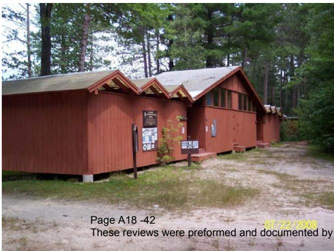
Bathhouse. By observation roofing and rafters have not changed since 2006 when it was recommended that deferred replacement and other maintenance be accomplished.
