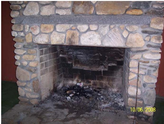
The group picnic area pavilion has damage to the firebrick in the fireplace and should be repaired by a professional mason. This pavilion also definitely needs a barbeque pit. The toilet building is adjacent. There is standing water by the swing set and pathway into the group area that could easily be removed with some simple drainage appurtenances.
