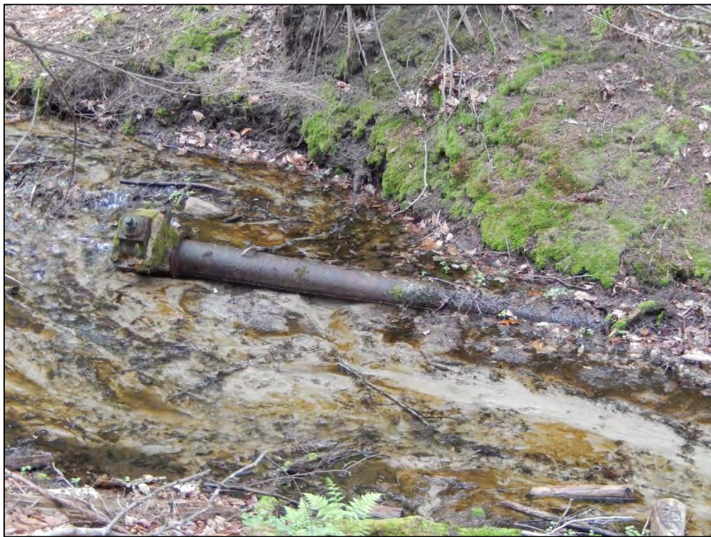
Figure 40. Steel pipe and valve near the location of the former fish hatchery.
