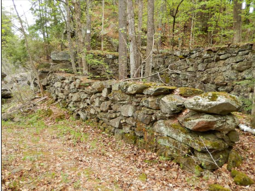
Figure 33. Fibreboard Company mill foundation 2, facing northwest.
