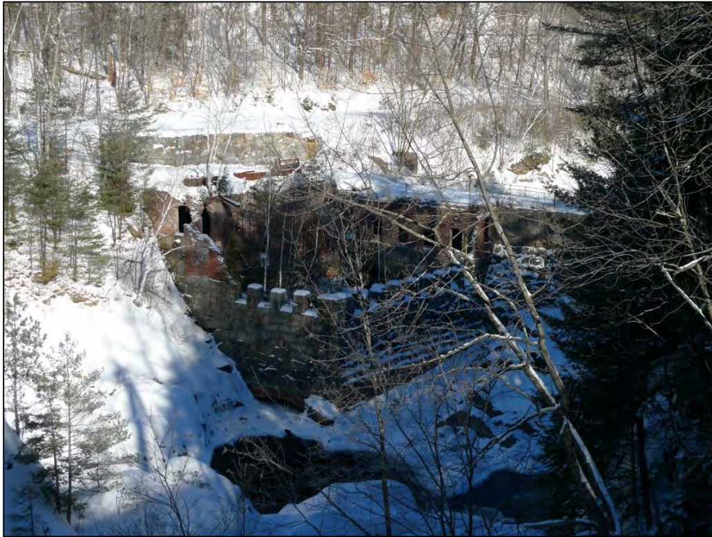
Figure 31. Foundation of the J. E. Henry and Sons pulp mill, facing northwest.
