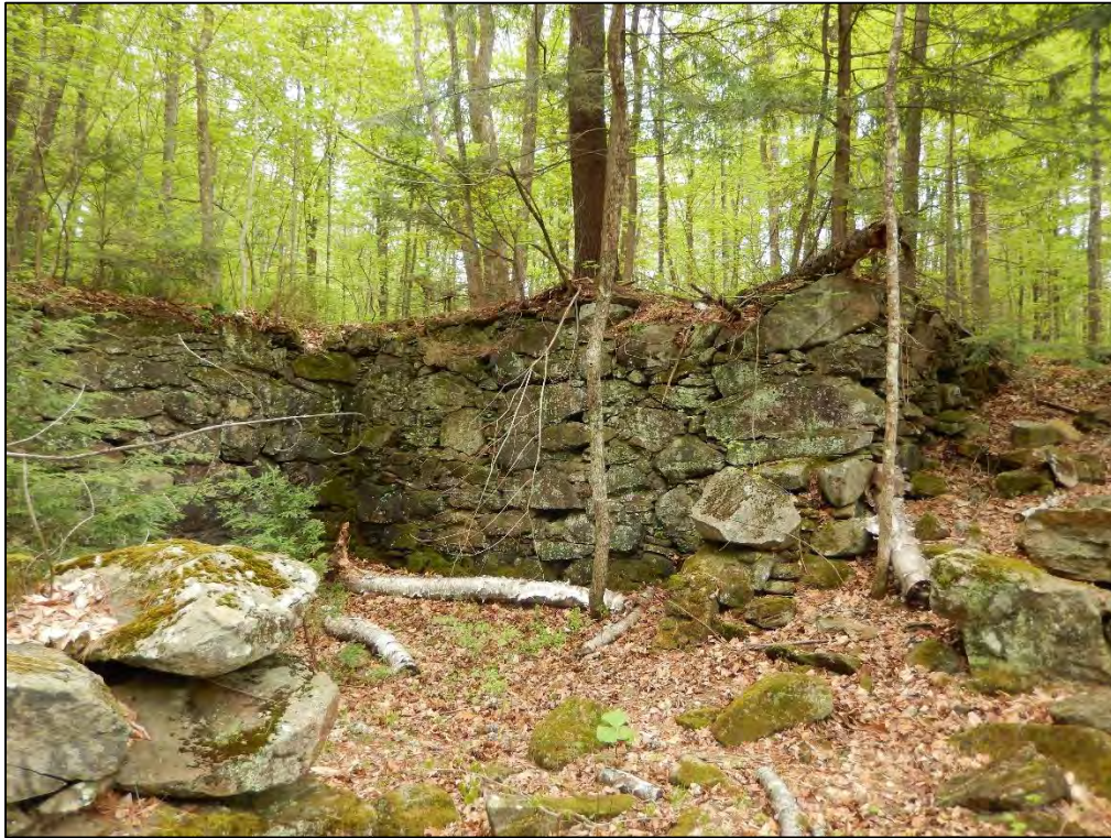
Figure 35. Fibreboard Company mill foundation, facing southeast.
