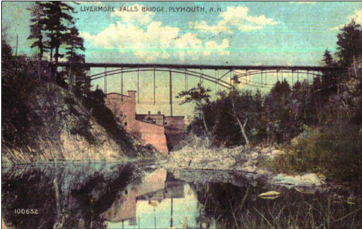
Figure 28. Pumpkinseed Bridge and the J. E. Henry and Sons pulp mill, ca. 1910.
