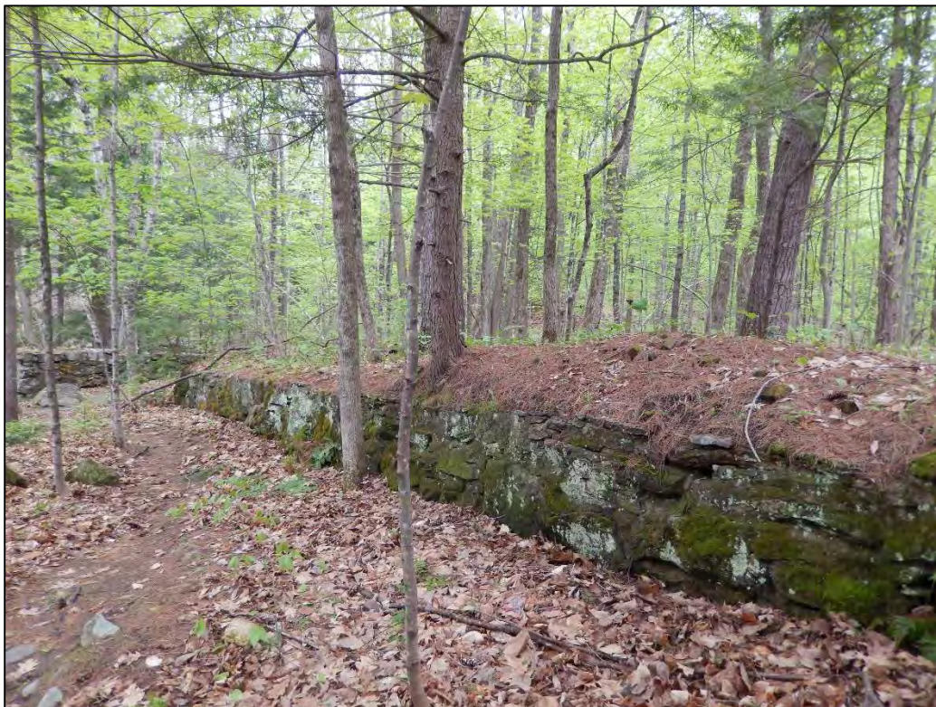
Figure 36. Eastern Lignoid Casket Company foundation, facing north.
