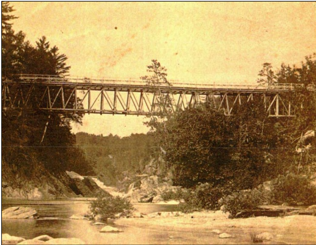
Figure 24. The wooden truss bridge prior to the pumpkin seed bridge, ca. 1875.
