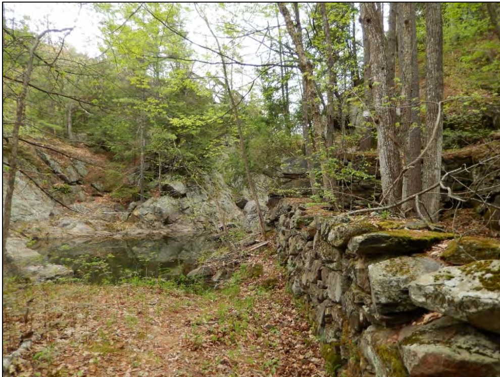
Figure 34. Fibreboard Company mill foundation 2, facing northwest toward site of former mill dam.
