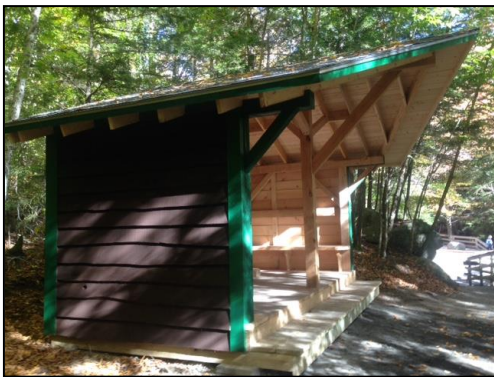
Top O' Gorge Rain Shelter Flume Gorge SP
