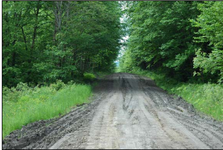
Figure 4.3: Wetness, poor road bed, and frost conditions contribute to rutting.
