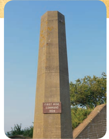
Stop #2 - a 3 story building surrounded this First Mine Command
