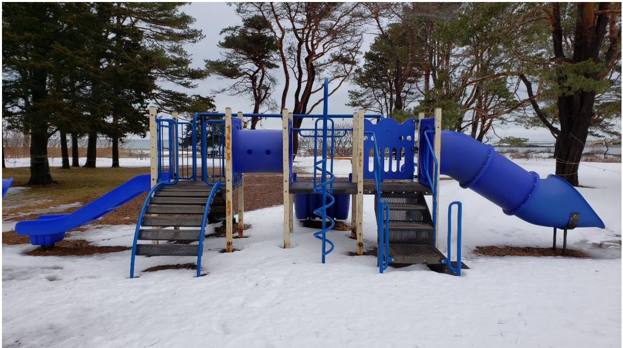
Remove and dispose the 2-5 playground structure (above ) and concrete footings
