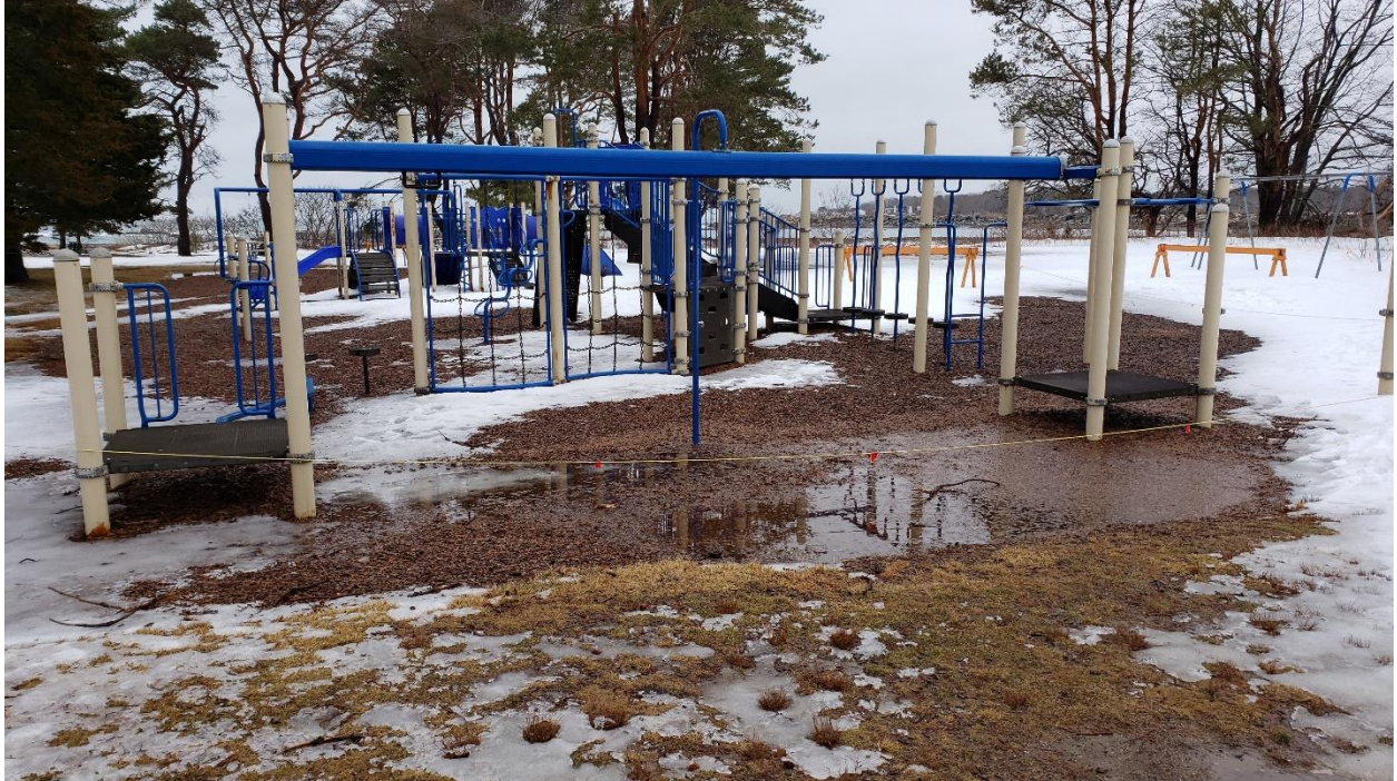
5-12 Structure Front 2-5 Structure middle 5" Arch Swing in background 3-leg swing set right
