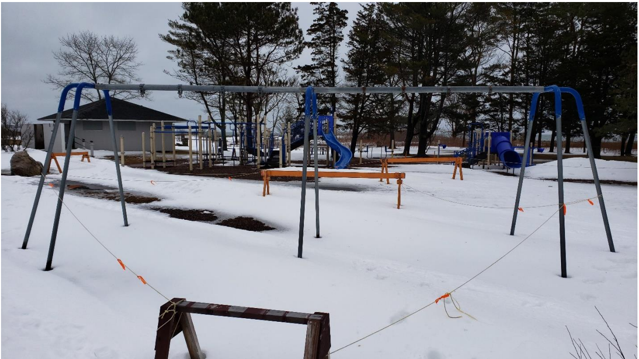
Remove the 2 bay swing (above) and concrete footings.
