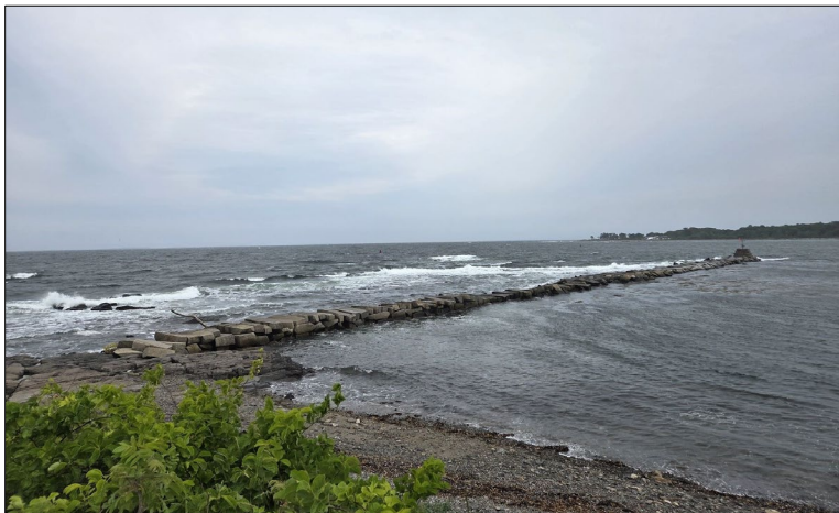
Photo: The breakwater between Little Harbor and the Gulf of Maine. Photo credit: Logan Spatola
