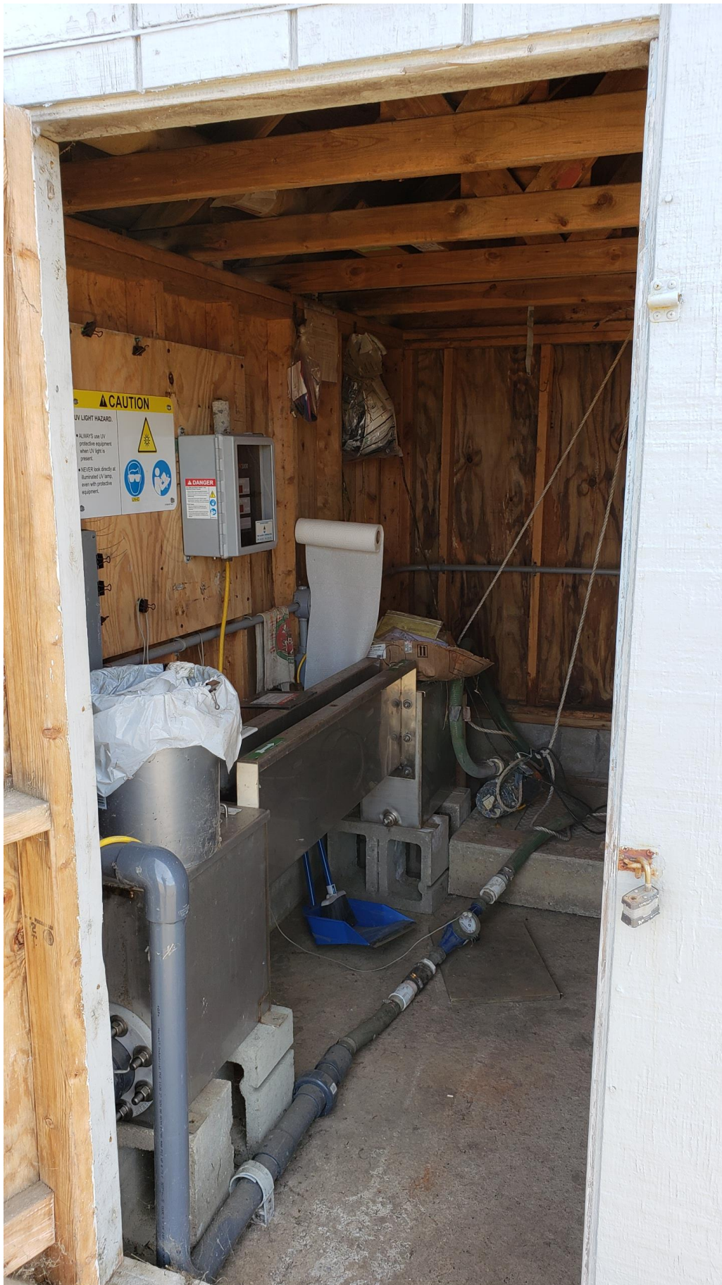
Trojan 3000 PTP UV Treatment System 5.
