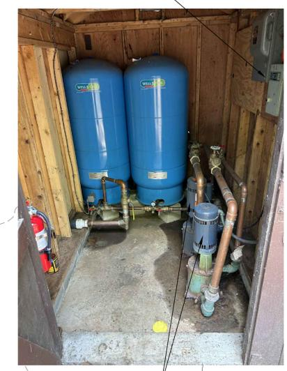
REMOVE AND REPLACE EXISTING PRESSURE PUMPS WITH NEW VFD BOOSTER PUMPS.
