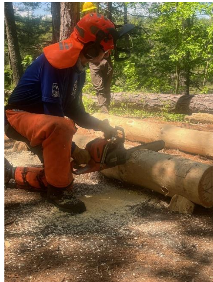
Timber Skills training in Brook State Park. A sawyer makes "kerf cuts" in a notch, which is then cleaned up with a chisel.
