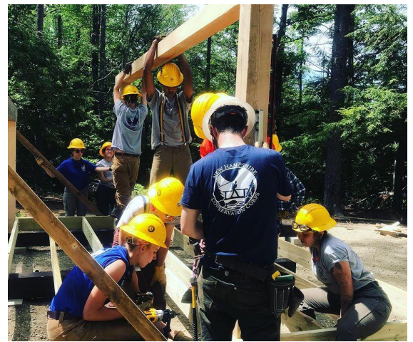
Carpentry Training at Greenfield State Park. Members construct the frame for a camping shelter.
