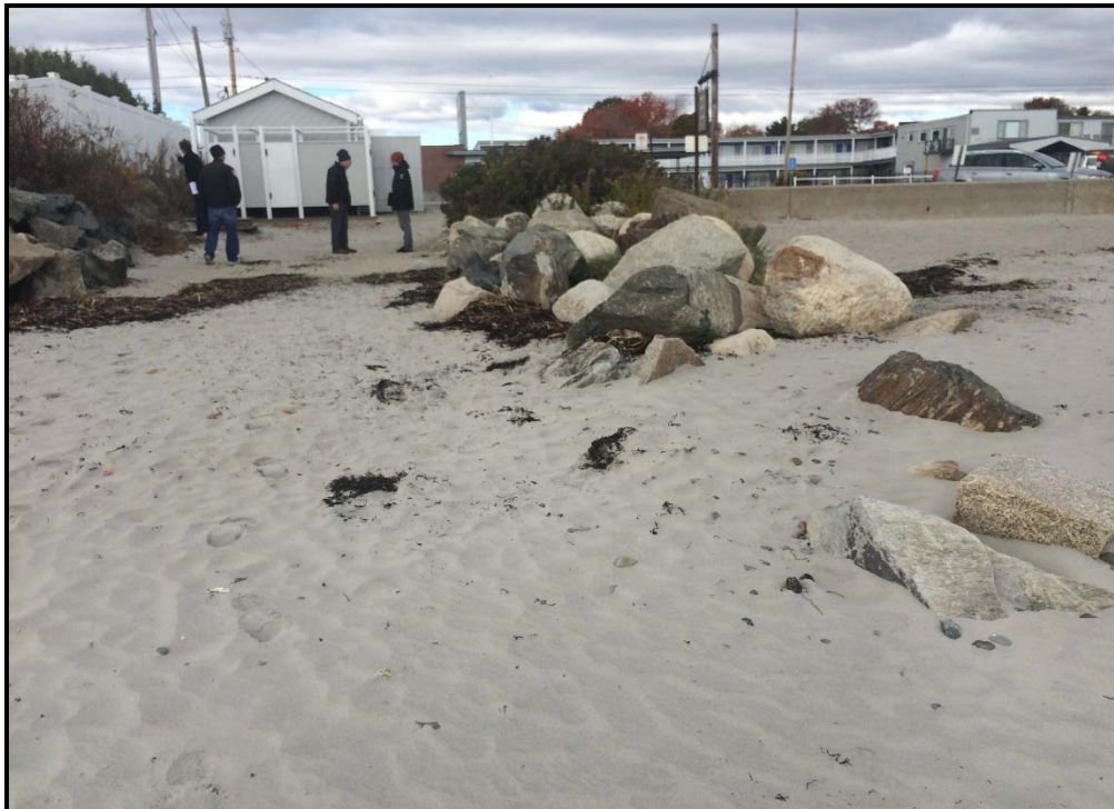
Photo 6: View west at the existing access path used by maintenance crews to access the beach with equipment and vehicles.
