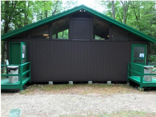
Newly Painted Bathhouse at Moose Brook SP
