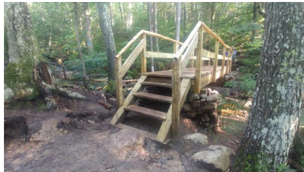
New Bridge on Arethusa Falls Trail, Crawford Notch SP
