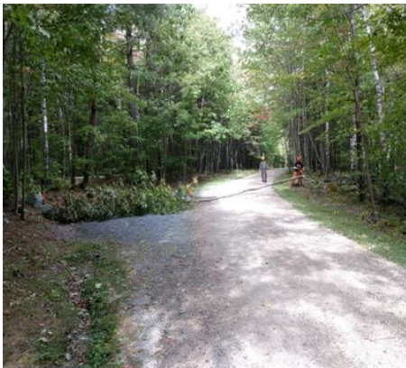
Felling trees to widen the road corridor at Mount Sunapee SP
