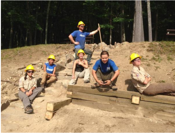
Posing on completed stone staircase and retaining wall at Silver Lake SP
