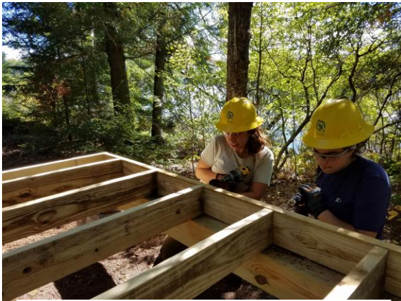
Constructing tent platform at Umbagog SP
