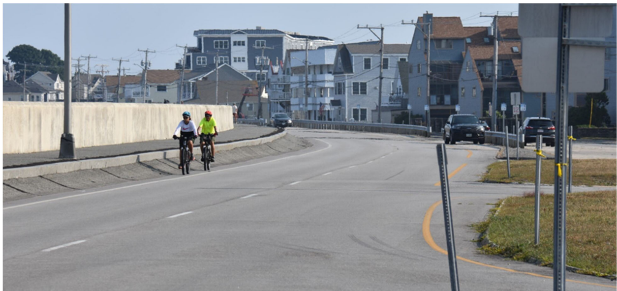
Figure 3-8. NH1A Excessive Grade Changes and Lack of Bicycle Accommodations
