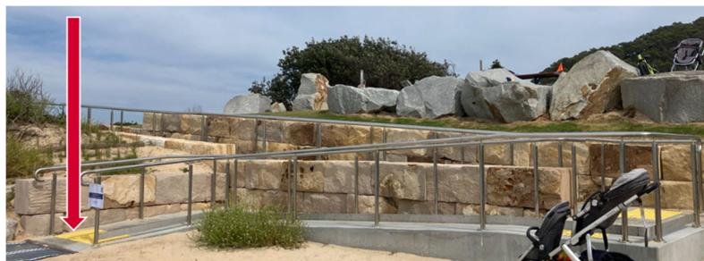
Figure 4-1. Tactile Paving Installation at Ramps
