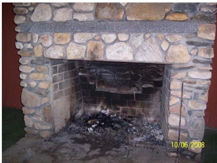
The group picnic area pavilion has damage to the firebrick in the fireplace and should be repaired by a professional mason. This pavilion also definitely needs a barbecue pit. The toilet building is adjacent. There is standing water by the swing set and pathway into the group area that could easily be removed with some simple drainage appurtenances.
