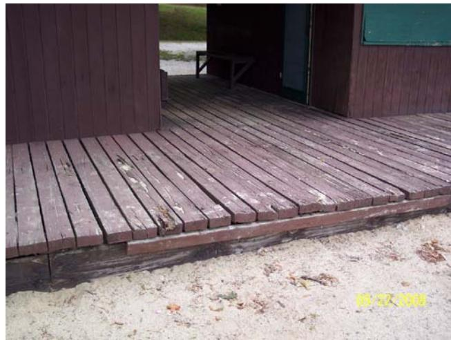
The walkway planking at the bathhouse and the store/office needs to be replaced. There are rodent holes and other pest infestations going on at the bathhouse. The old playground swing set shows plenty of use and that area could be maintained better, as should the horseshoe pits. The 0.3 mile nature trail is an amenity if interpreted.
