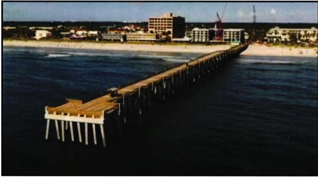
Jacksonville Beach Pier (Image from Internet - Credit: EMT)
