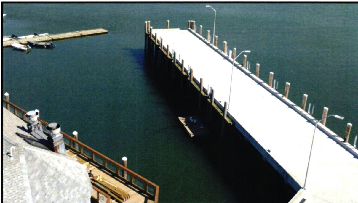
Angled Pier with Concrete Deck (GEI Project Example)
