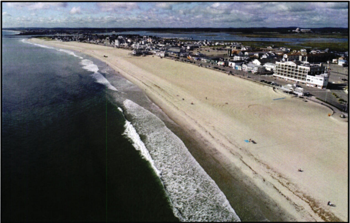
Pier Location Area 2 (Middle) Looking South
