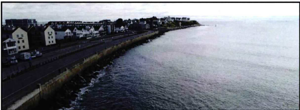
Pier Location Area 1 (North End) Looking at East at Boars Head
