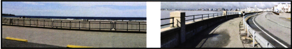
Seawall At Middle of Beach
