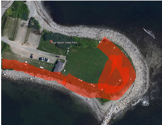
Debris removal area highlighted in RED
